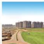
Construction in full swing
