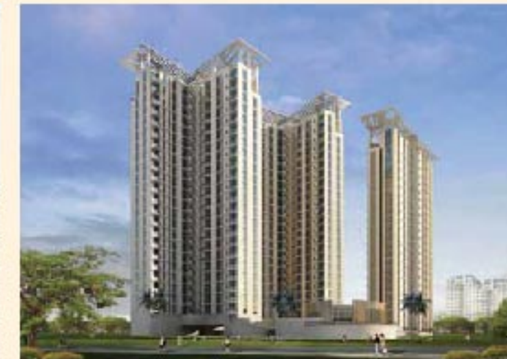
Swarnamani Canal Circular Road, EM Bypass, Kolkata
