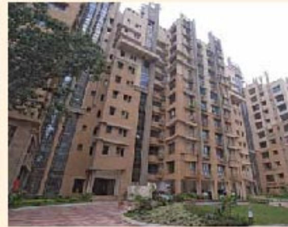
Mani Karn Opp. Salt Lake Stadium, on EM Bypass, Kolkata
